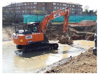
Figure 9: Photo showing mixing the reagent into the top layer of material using a specialist attachment on the arm of the excavator.
