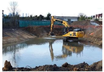
Figure 7: Photo showing that the depth of the dig was just beneath the groundwater level to reduce over-excavation.
