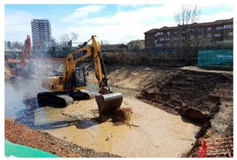
Figure 8: Photo showing the excavator adding the oxygenating compound. The machine used for subsequent mixing is seen in the background.
