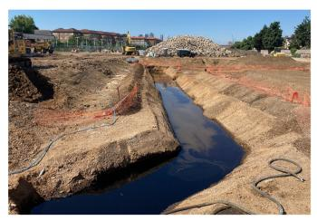
Figure 6: Recovery trench constructed in north eastern source area.
