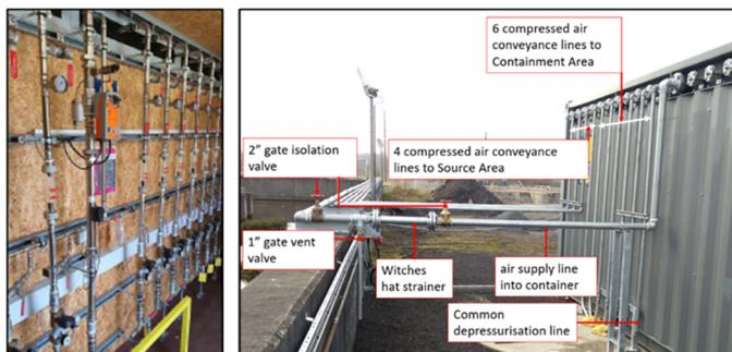
Figure 7: Biosparge system manifold and air supply conveyance pipes.
