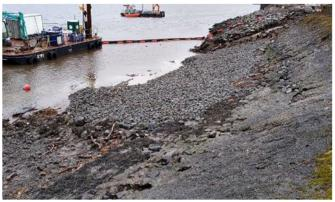
Figure 9: Area of filter stone placement.
