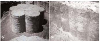
Fig 2. Examples of constructed columns using soil mixing augers: (a) overlapping configuration and (b) barrier wall configuration.
