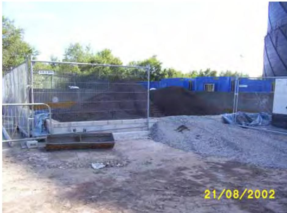
Plate 6.3: Completed soil-holding pen with soil feedstock in place and security fencing
