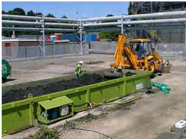
Plate 2.1: A mobile landfarm being operated at a gasworks in northern England.
