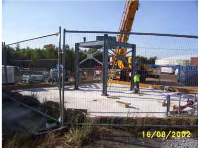
Plate 6.4: Bioreactor frame in position in the bioreactor compound
