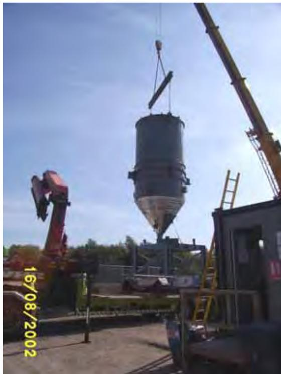
Plate 6.5: Lifting the vessel of the bioreactor into the frame
