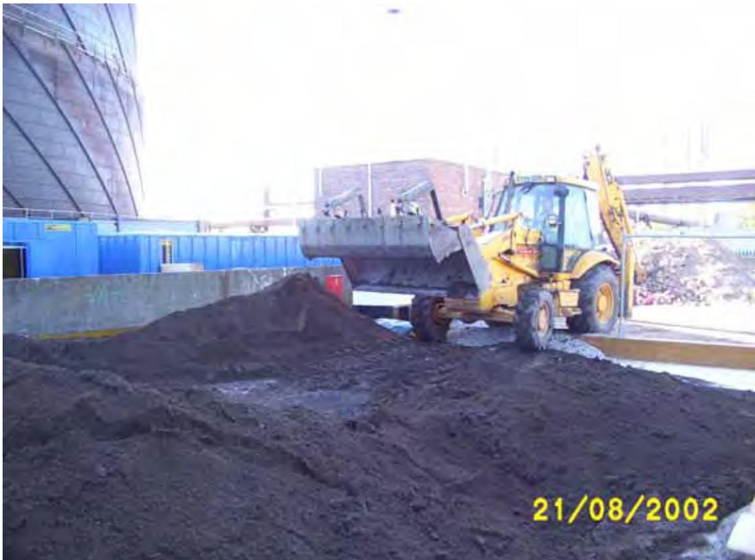
Plate 6.15: JCB mixing the coal tar recovered from the tar tanks with soil from the site. Tar to soil ratio was approximately 1:3
