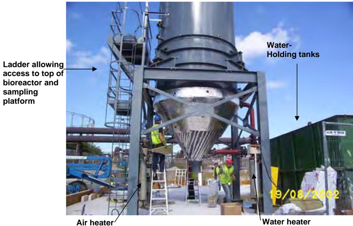
Plate 6.6: Installation of lagging over the trace heating system
