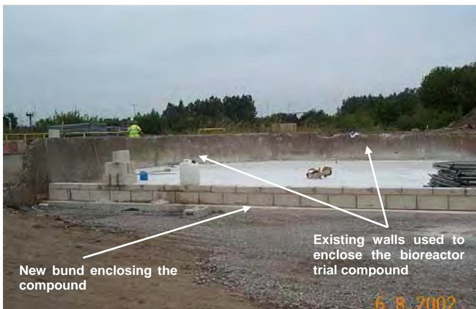
Plate 6.1: Bioreactor trial compound prior to waterproofing the concrete walls and breezeblock bund
