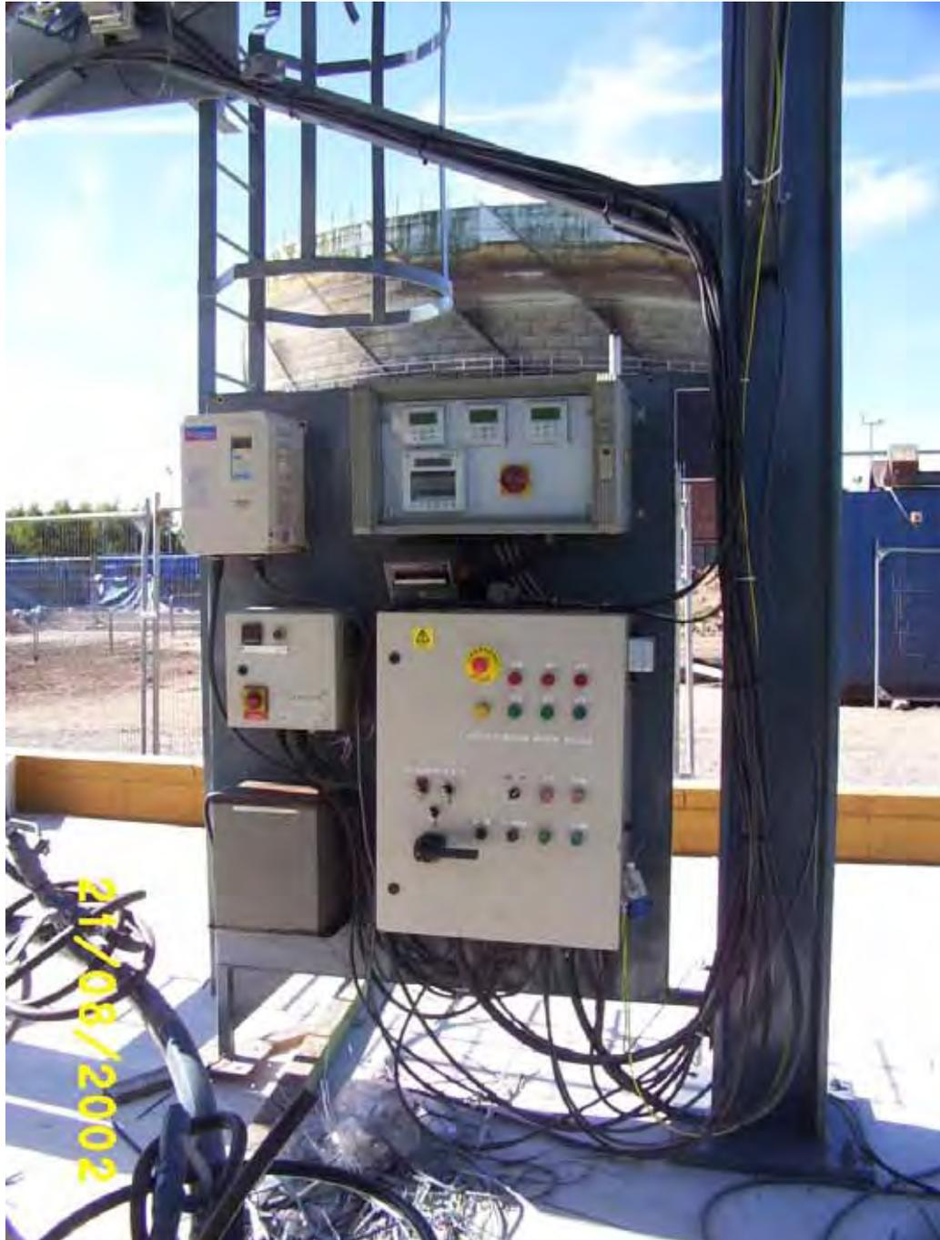
Plate 6.11: Main control panel and electrical connections (including telemetry field bus)
