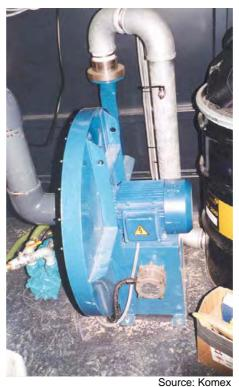
Plate 7.5: Soil vapour extraction pump
