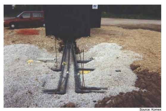
Plate 7.7: All pipework entering unit from below
