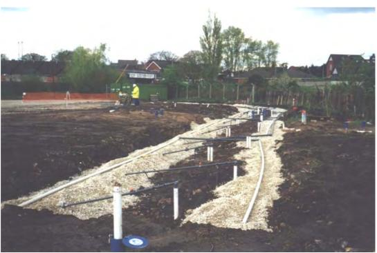
Plate 7.2: SVE extraction pipework laid horizontally
