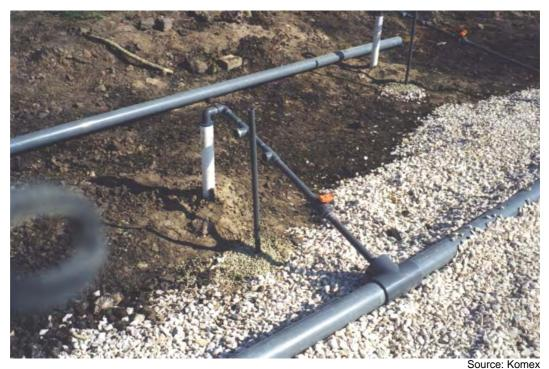
Plate 7.1: Air injection pipework connected to wellhead
