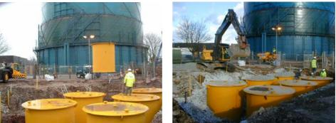
Plate 6.1: Sequential images of the installation process of the SEREBAR: a) excavation of the cut-off trench, b) installation of a deep well downgradient of the reactive gate, c) lifting canisters into position, and d) backfilling space around canisters
