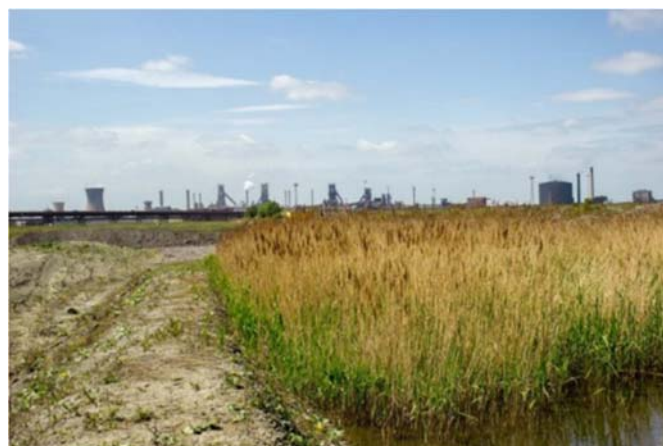
Figure 5: Pilot reedbed dominated by Common Reed ( Phragmites australis ) treating alkaline (up to pH 12) leachate at Scunthorpe
