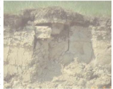
Figure 7. Damaged compacted clay cover system in southern Wisconsin caused by desiccation (Benson, 1999).
