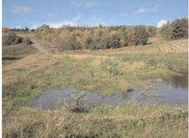
A REDUCING AND ALKALINITY PRODUCING SYSTEM (RAPS) FOR PASSIVE TREATMENT OF ACIDIC, ALUMINIUM RICH MINE WATERS
