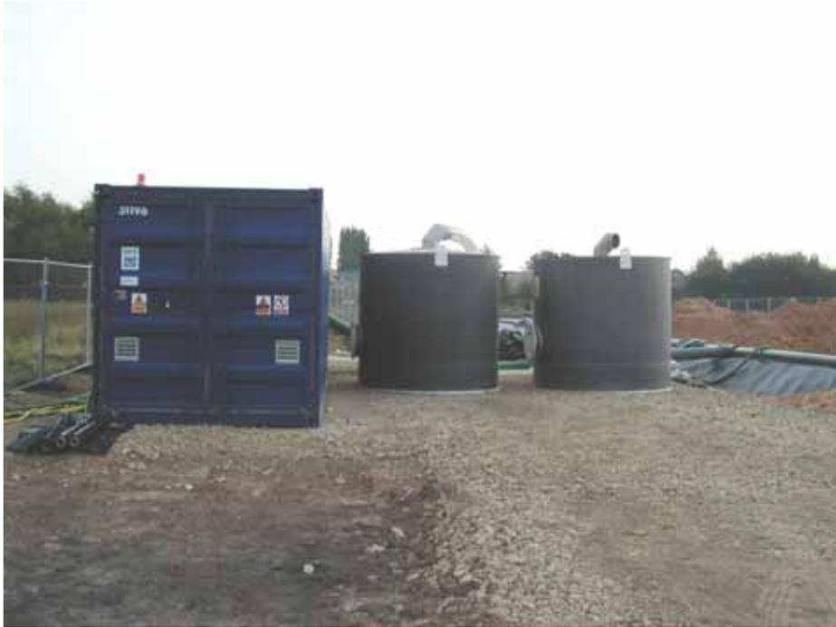
Plate 7.5: Container Housing Vacuum Pumps and Activated Carbon Vessels.
