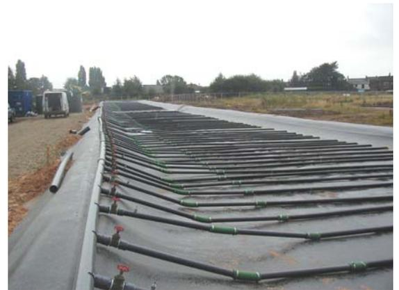
High density polyethylene liner and vapour extraction pipe array
