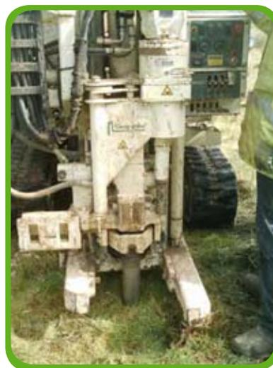
Figure 3.2: Drilling of boreholes (part of the Site Investigation)
