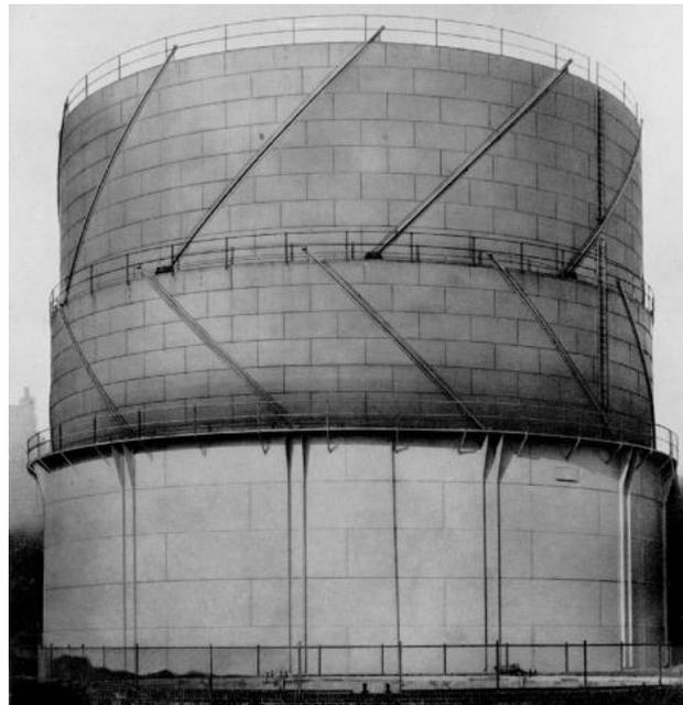
**Photograph 7. Spiral-guided gasholder with two lifts in a steel above-ground tank.**
