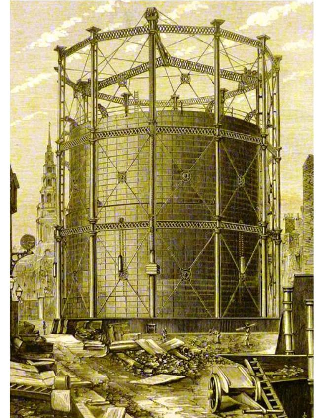
Figure 7. A three-lift column-guided gasholder at the City of London Gas Company's works at Blackfriars, London. From King's Treatise, Vol II, 1879.
