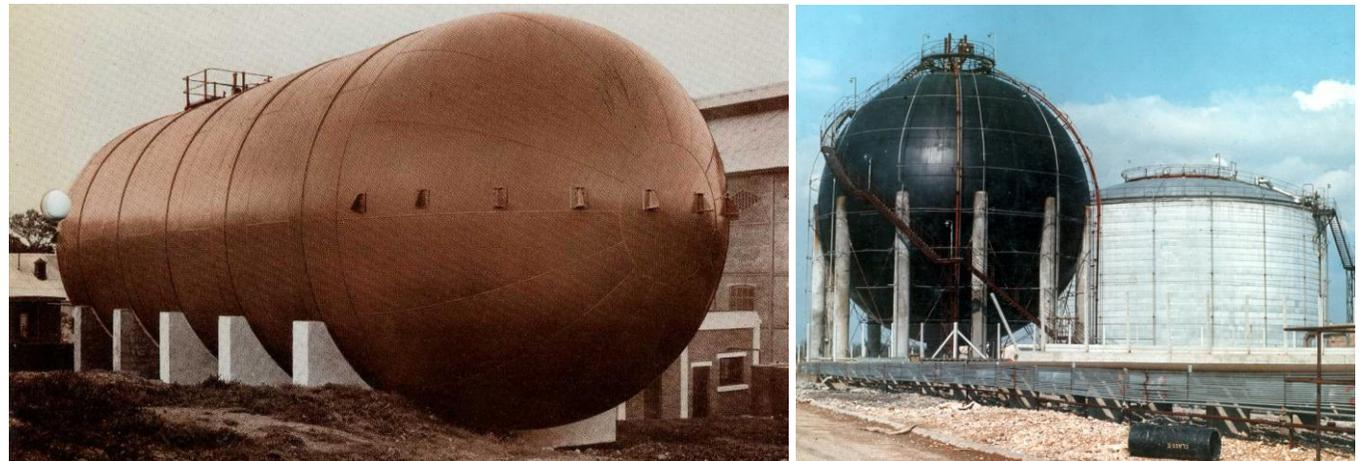
**Photograph 4. A high-pressure bullet-type gasholder (left, courtesy of the IGEM PHI) and high pressure sphere gasholder (right), behind which is a small LPG tank.**
