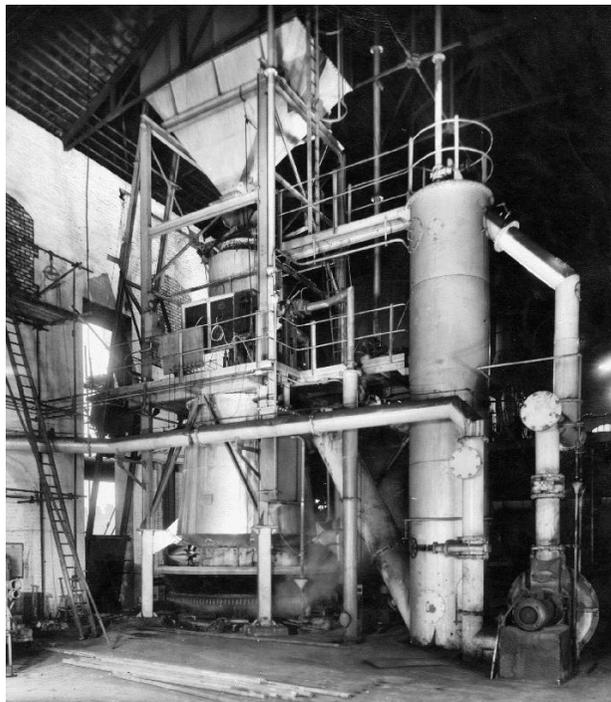
**Photograph 6. Gas producer (left) and Scrubber (right) at the former Garston gasworks, 1947. Source: National Grid Gas Archive.**
