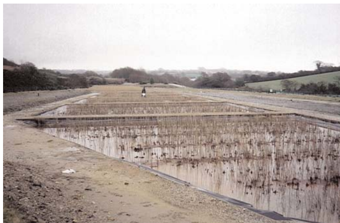
Figure 5: Growth of the introduced reed species in the lime dosed system compared to luxuriant growth in the aerobic cells of the ALD system in the background. Source: G.Hall
