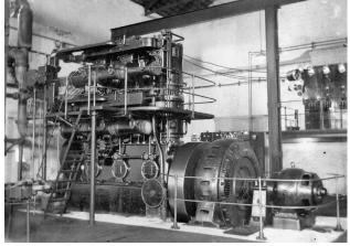
Photograph 5. Gas engine powering an electrical generator at a colliery powerhouse, 1914. Source: National Grid Gas Archive.
