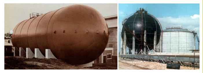
Photograph 4. A high-pressure bullet-type gasholder (left, courtesy of the IGEM PHI) and high pressure sphere gasholder (right), behind which is a small LPG tank.
