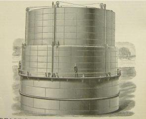
**PEASE'S PATENT WIRE ROPE GUIDING** Figure 8. A cable-guided gasholder in an above-ground steel tank. From an old advert *circa* 1880.
