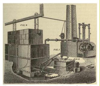
Figure 2. The gasworks built by Clegg for Ackerman, a famous London printer, indicating the retort setting (Fig.1), tar receiver (Fig.2), lime purifier (Fig.3) and gasholder (Fig.4). From the Journal of Gas Lighting.
