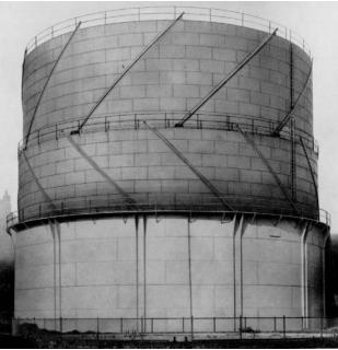
Photograph 7. Spiral-guided gasholder with two lifts in a steel above-ground tank. Source: IGEM PHI.
