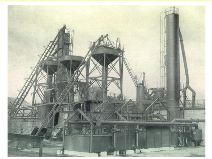
Photograph 8. A producer gas plant with cooling and purifying plant for gasification of bituminous coal. Source: National Grid Gas Archive.
