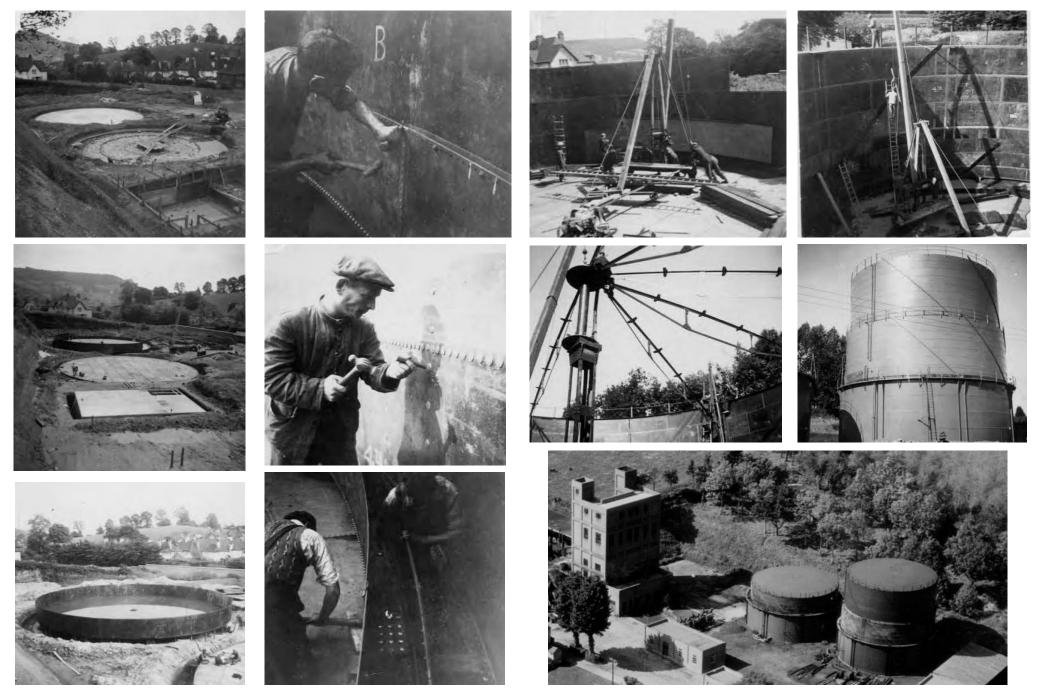
Photograph 16. Construction of two above-ground spiral-guided gasholders at a former gasworks in South-West England. Source: IGEM PHI.
