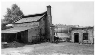
Photograph 15. A typical village gasworks in Somerton, Somerset. The main building is the retort house, the gasholder can be seen behind.
