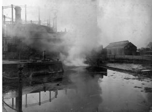
Photograph 53. Running off pitch into pitch beds.
