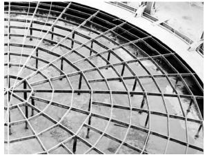
Photograph 10. A gasholder with the sheeting removed from the crown, exposing the crown rest and water-filled tank.
