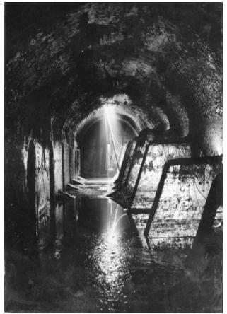
Photograph 43. Interior of a tar tank at the former gasworks, Sydenham.
