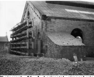
Photograph 24. A horizontal atmospheric condenser.
