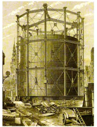
Figure 7. A three-lift column-guided gasholder at the City of London Gas Compan's works at Blackfriars, London. From King's Treatise, Vol II, 1879.
