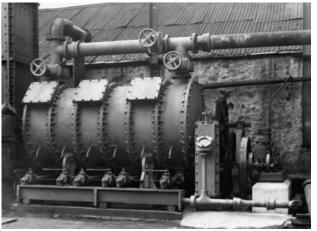
Photograph 32. A rotary mechanical washer.
