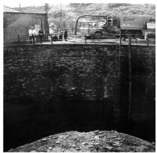
Photograph 11. A brick gasholder tank with dumpling visible at the base.
