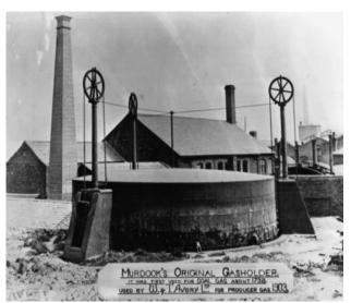
Photograph 4. Murdoch's original circular gasholder at the Soho works.
