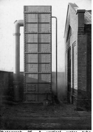
Photograph 25. A vertical water tube condenser.
