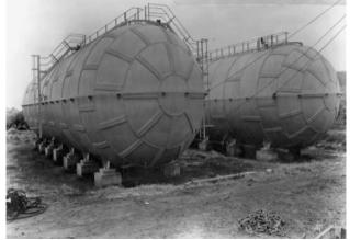
Photograph 41. High-pressure bullet tanks.
