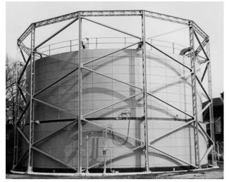
Photograph 5. A two-lift frame-guided gasholder with below-ground tank, using Cutler's patented system, Southern England. Source: IGEM PHI.
