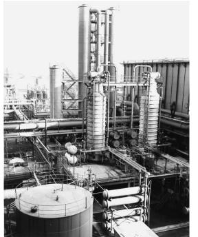
Photograph 47. Large benzole plant at the former Carr House gasworks in Rotherham.
