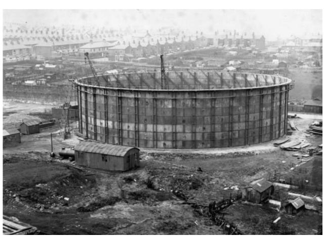
Photograph 15. Construction of an above-ground steel tank.
