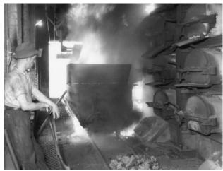
Photograph 20. Unloading a through-ended retort mechanically.
