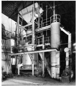
Photograph 6. Gas producer (left) and Scrubber (right) at the former Garston gasworks, 1947. Source: National Grid Gas Archive.
