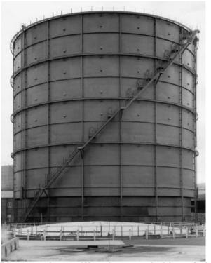
Photograph 40. Waterless gasholder of the Wiggins design.
