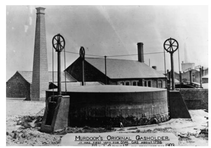
Photograph 3. The primitive gasholder at the first small gasworks at the Soho factory of Bolton and Watt.
