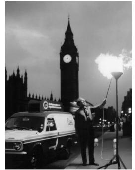
Photograph 13. The Conversion Programme. Flaring off town gas from the gas mains.
