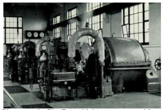
Photograph 52. Four high-pressure turbinedriven boosters at the former Beckton gasworks.
