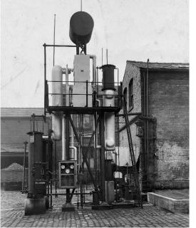
Photograph 46. A small benzole plant at the former gasworks in Middleton.
