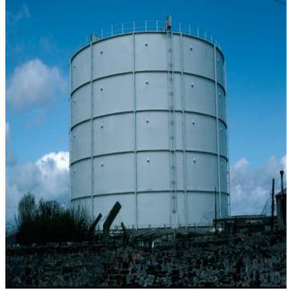
Photograph 9. Wiggins type gasholder at Millom, England. Source: Mr Syd Bennet.
