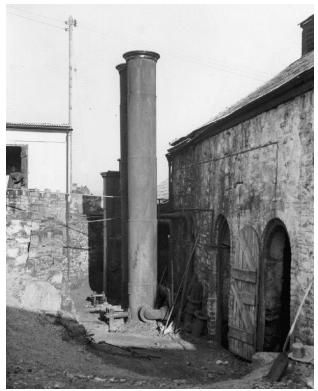
Photograph 23. A set of two atmospheric condensers, Gunnislake gasworks, Cornwall.
