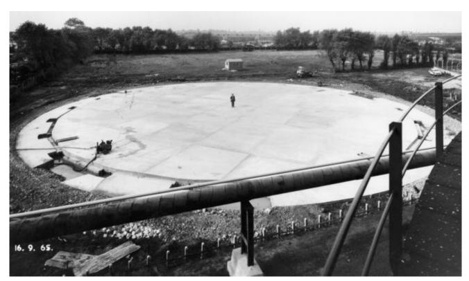
Photograph 12. Concrete foundation slab of an above-ground gasholder.
