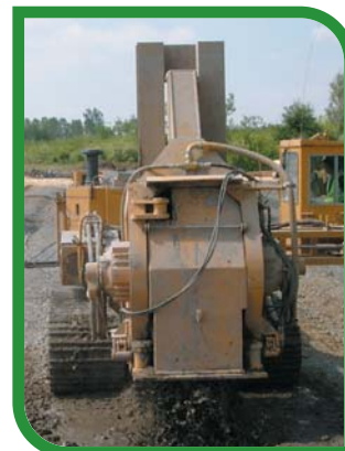
Various Perspectives of SMT in Progress Using 'Trenchmix'
