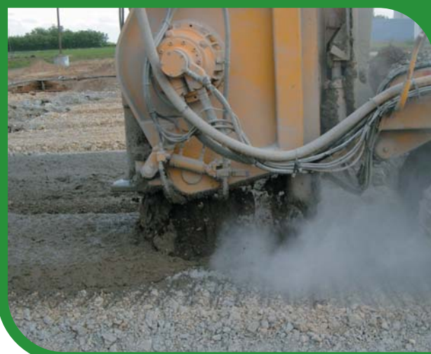
Soil Treatment for Grape Storage Facility, France
