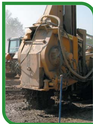
Various Perspectives of SMT in Progress Using 'Trenchmix'
